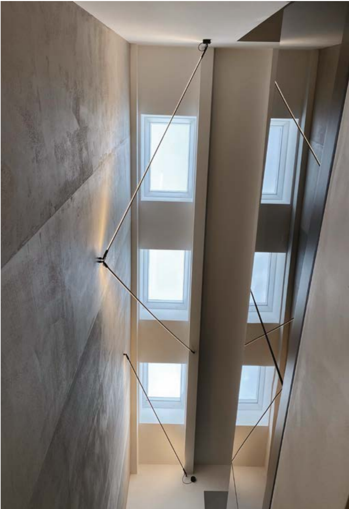
Special installation with remote driver and pass-through connection between two profiles.
